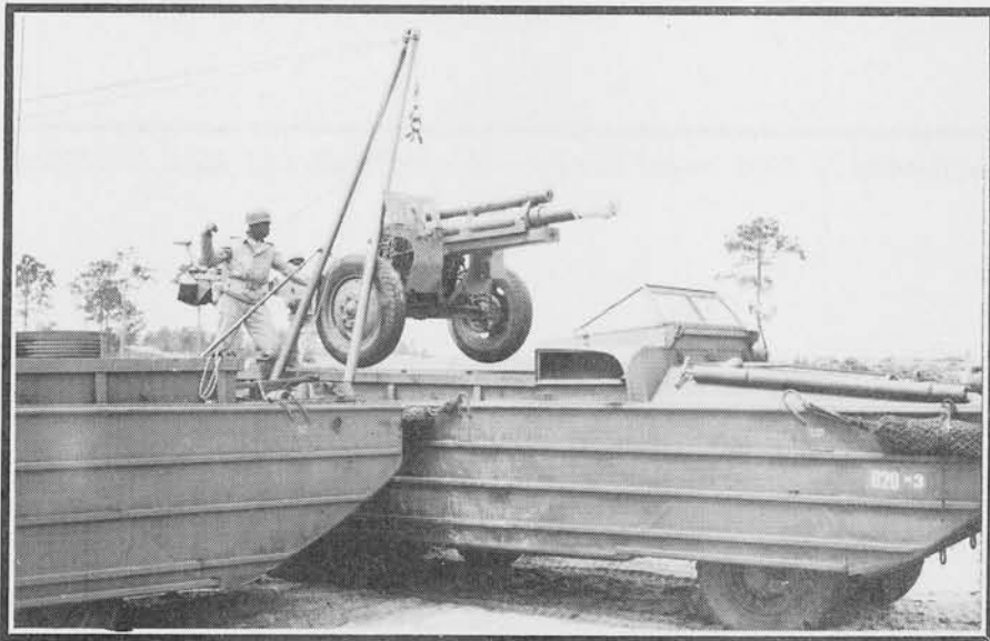
Unloading a 105MM Howitzer with "A" Frame
