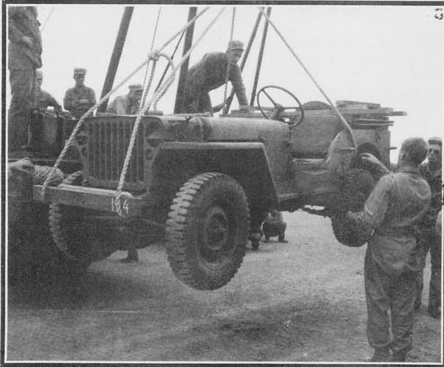
Lifting a Jeep with an "A" Frame.
