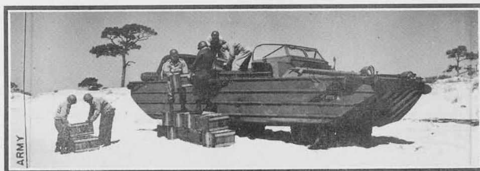
Hand Unloading Platform
